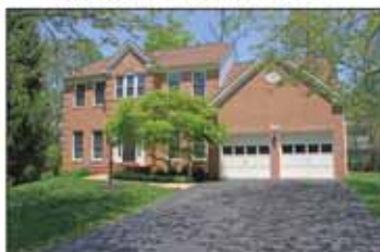
Arcadian Shore Court
